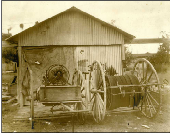
Original fire station in use 1914 to 1921 This is the first fire fighting equipment ordered for the town by George E. Sebring.
