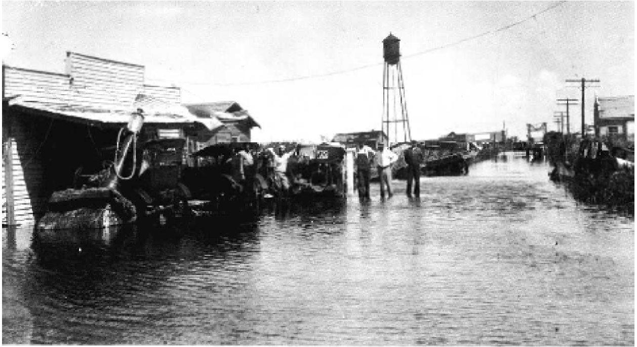
Main Street of Moore Haven after the flood had receded following the September 1926 Hurricane
